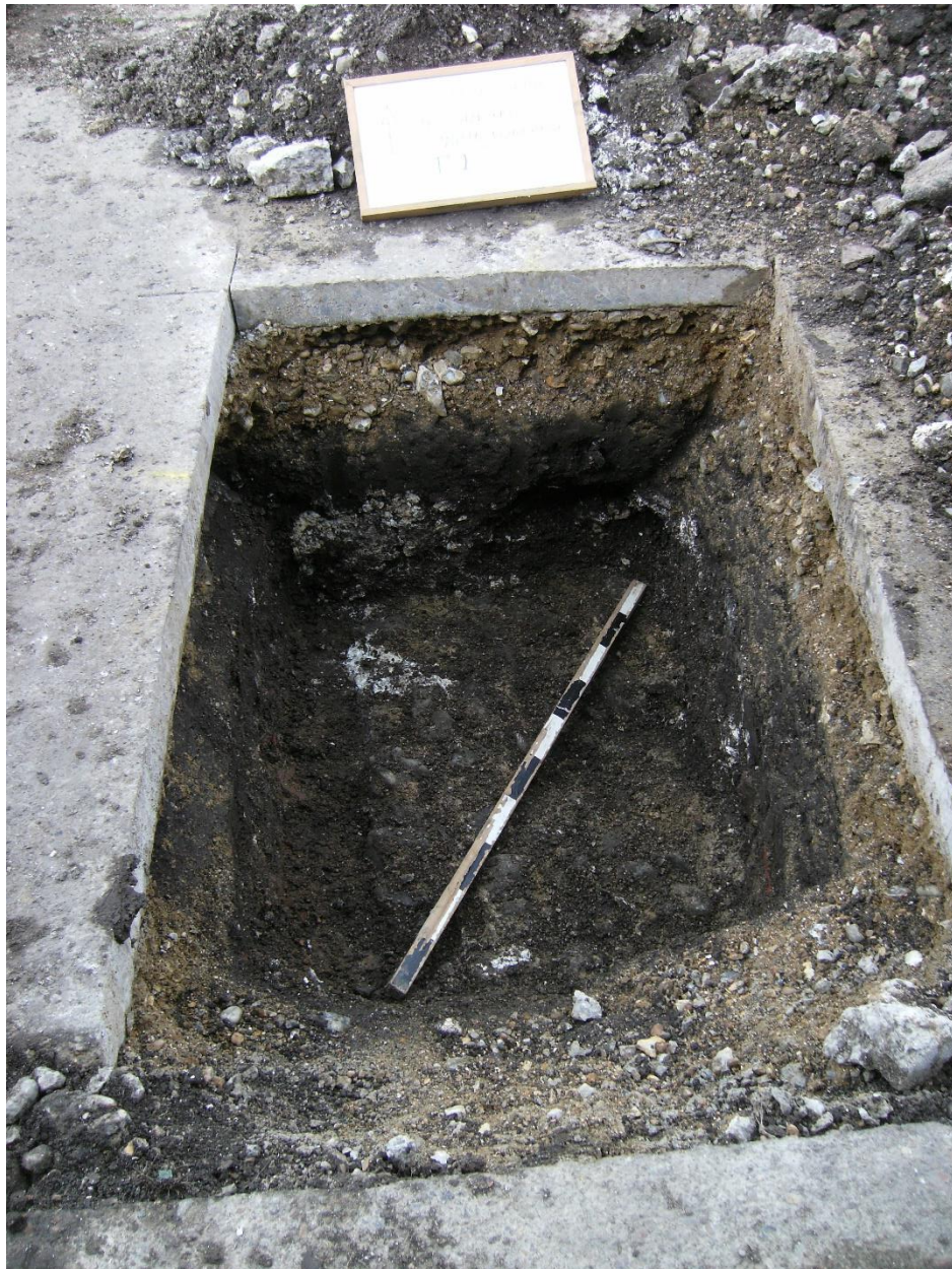
Plate 18. Test pit 22 from the south showing the western wall foundation of the Common Hall exposed at its base, one-metre scale
