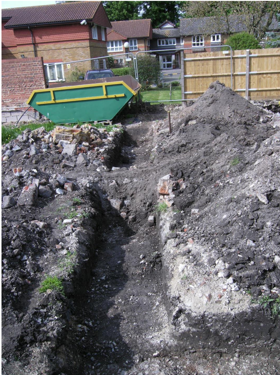
Plate 23. The trench following the removal of topsoil and prior to the excavation of test pits 17, 18, 19 and 20, looking north
